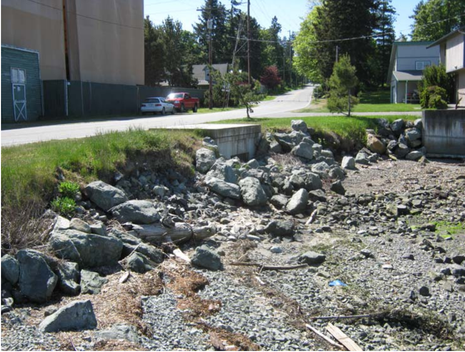
Photo 8. Holmes Harbor shoreline adjacent to Shoreview Drive. Looking west.
